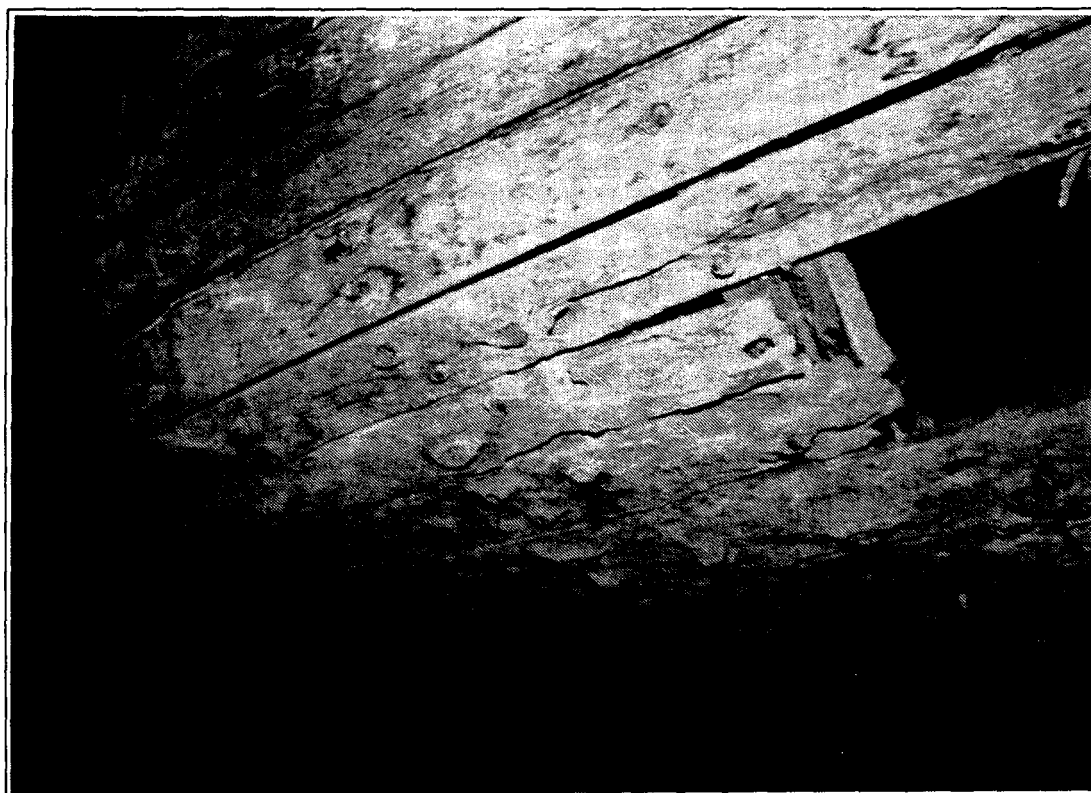
Figure 6 Hull planking on the P.S. Colonel.
